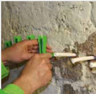
Installation of the KÖSTER Capillary Rods and KÖSTER Suction Angles
