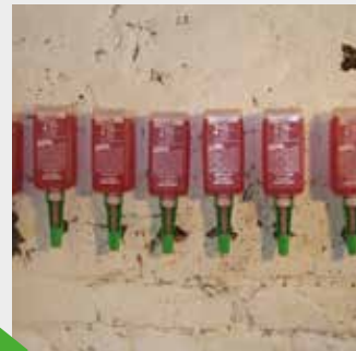
Automatic installation of the horizontal barrier
