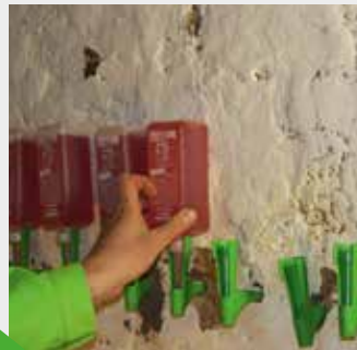
Installation of the cartridges
