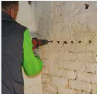
Horizontal drilling in the bed joint
