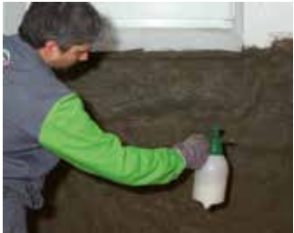
Priming with KÖSTER Polysil TG 500
